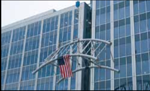
Final piece of tiara lifted into place, July 2010
